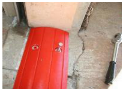
Fixing anchors into concrete
