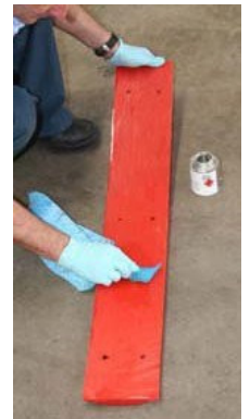
Cleaning the bund underside
