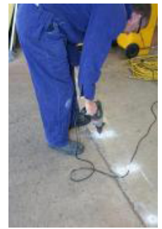
Drilling holes in the concrete
