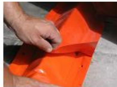
12. To make a join, cut off excess PVC to the end of the foam on one of the pieces. Cover the areas to be adhered with glue. Insert cut off end into end with excess PVC (you may need to pull welds apart to 150mm and cut off 150mm of foam) and press surfaces together when tacky.
