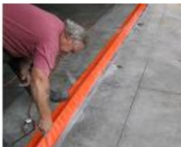
14. Repeat steps 1-10 when joining the other end of the bunding to the wall and finish bolting down the side away from potential spills. An additional hole may be required to be drilled in the aluminium strips to ensure the bunding is secure at the ends and at the corners.
