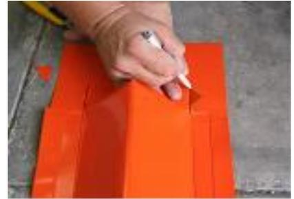
3. Fold flaps over the face of the foam. Mark and cut away excess in line with the side welds.
