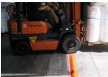
16. Finish by running a bead of Sikaflex along the joins to the wall. Allow 12 hours to cure before driving over your new bunding
