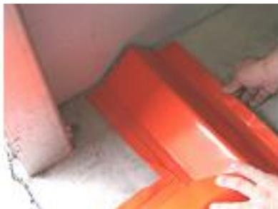
13. Continue to bolt down aluminium strips on the side away from the potential spill.
