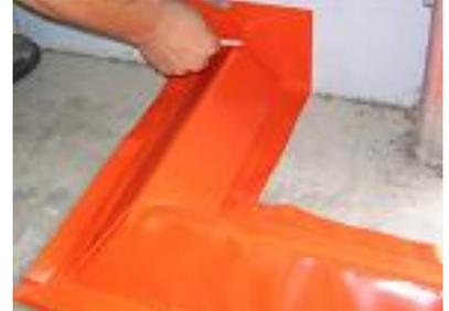
6. Fold bottom flap up and push end up against the wall. Mark bunding profile on the folded up bottom flap.
