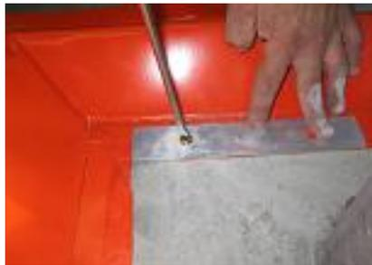
11. Using holes in the aluminium strip as a guide, drill concrete and bolt aluminium down using the masonry anchors on the side facing away from the potential spill.
