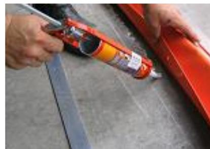
15. Run a bead of Sikaflex between the bunding and the ground one length of aluminium at a time. Bolt aluminium strip down. An additional hole may be required to be drilled in the aluminium strips to ensure the bunding is secure at the ends and at the corners.
