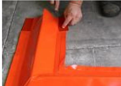
2. Remove excess PVC material from the sides of the top flap only.
