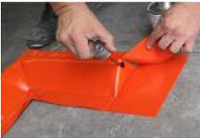
4. Fold one flap under the foam. Apply glue to the front of the folded flap and the back of the remaining flap.
